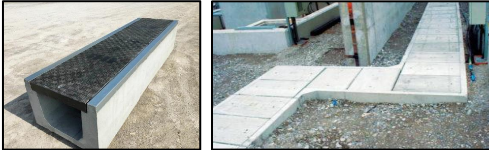
Fig 7.17(a): A concrete duct with removable lid and duct installed in a substation Applications:
