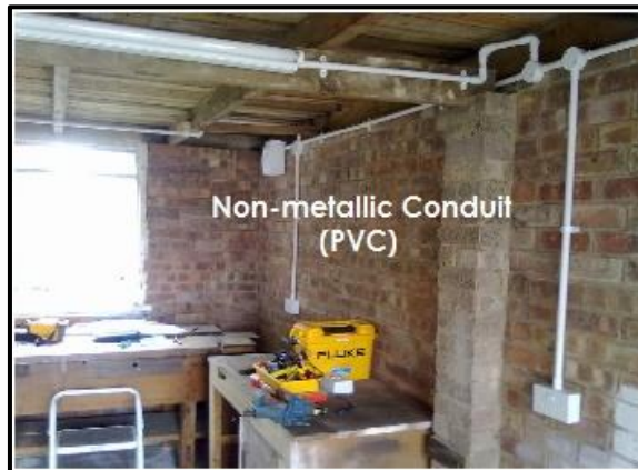
Fig 3.1: Surface type PVC conduit wiring system
