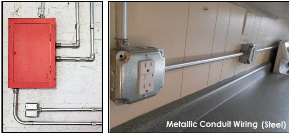
Fig 7.1: Steel conduit wiring system
