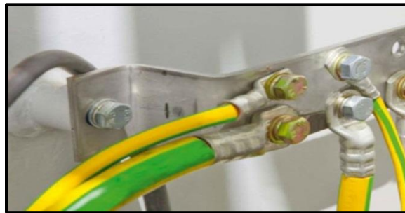
Fig. 4.9: Earth plate and connections of earthing lead and earth continuity conductors
