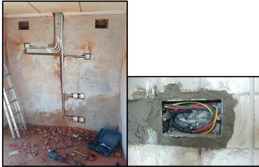
Fig 3.6: Grooves in brick wall for concealed conduit/boards installation
