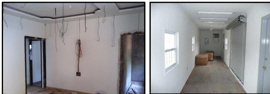
Fig 3.4: Concealed conduit wiring under construction (left) and after finish (right)
