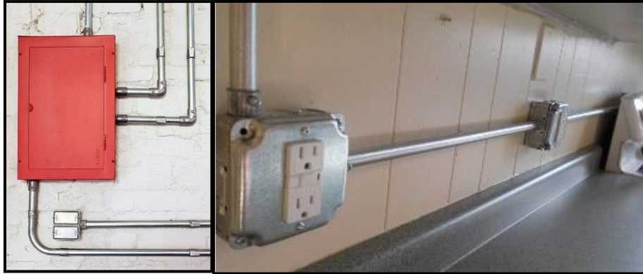
Fig 3.7: Surface steel conduit installation
